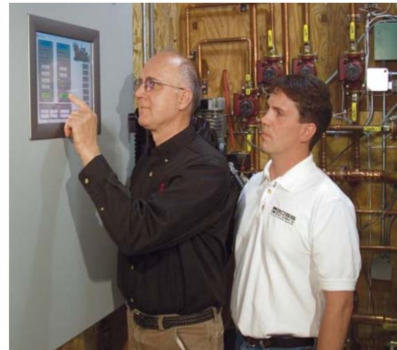
"The new system is able to hold the temperature dead-on, with variations inside the room at less than one degree from floor to ceiling, and humidity is stable as set." (left to right) Gordon Vadis (BugCo), Mark Antczak (BOSS Control Systems)
